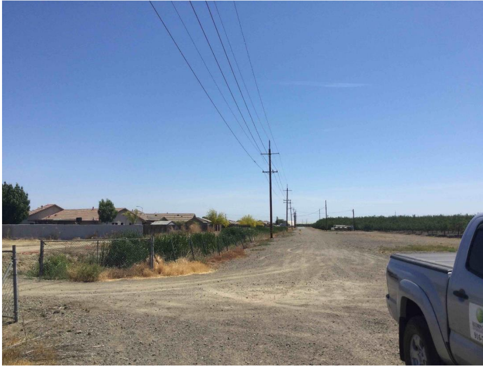
Photo 1: Roadside ditch and existing electrical power line along Husted Lateral Road
