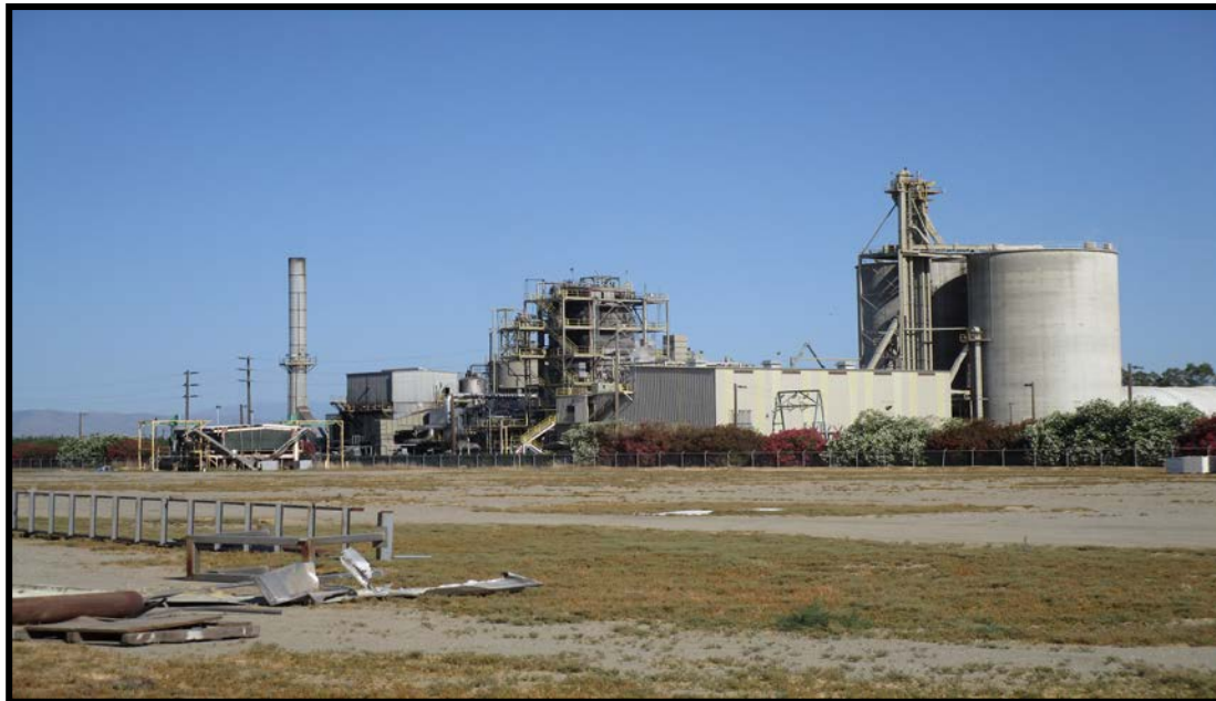
Exhibit 5 – Property to the North (Wadham Facility)
